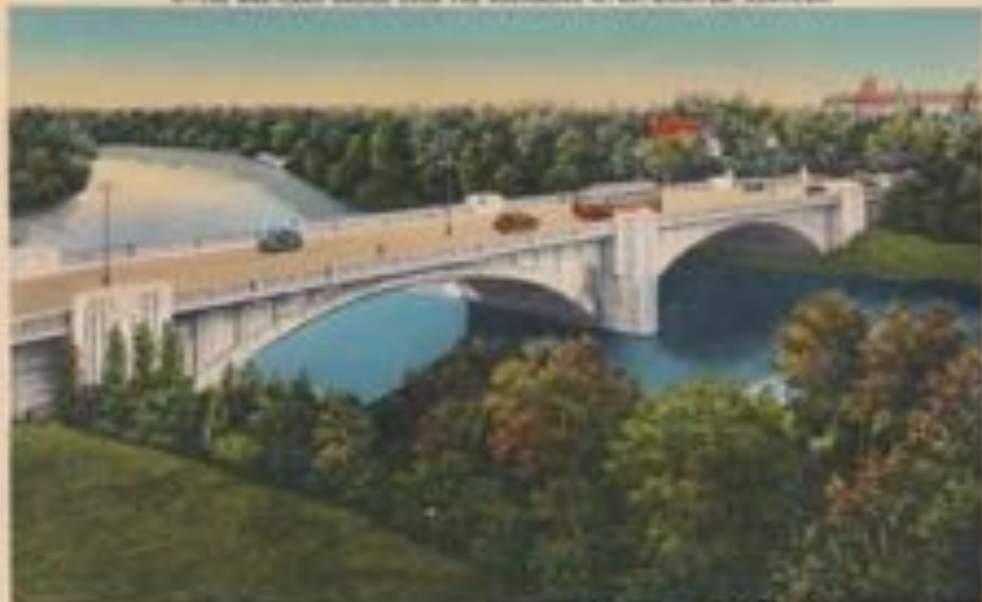
17—THE WYPLAND BRIDGE OVER THE ABBINGTON RIVER, WINDFEL, SAUTTER.
