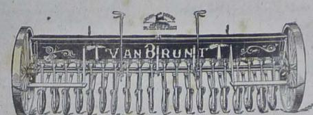
Van BRUNT Light Draft Grain Drills owe their success to their practical working qualities. They were the first to overcome all objections on account of clogging, chocking up or poor seeding, and can be depended upon for working in mud, corn-stalks or trachy ground, as well as in clear, dry soil.
