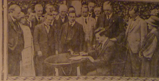
Though Australia's new federal capital, Canberra, in New South Wales, is only just begun, the federal cabinet recently held its first meeting there. This photograph shows the acting prime minister signing the first document in the open air because no building is yet completed.
