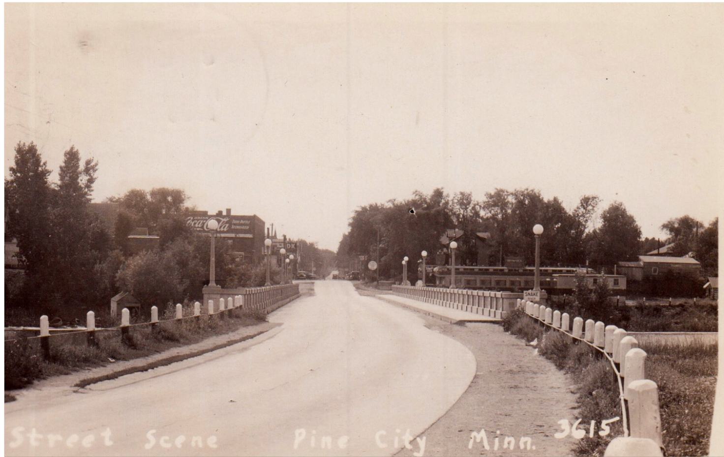
This photo was taken about 1940. Looking south you can see Brownies Cafe on the southwest corner of the bridge.
